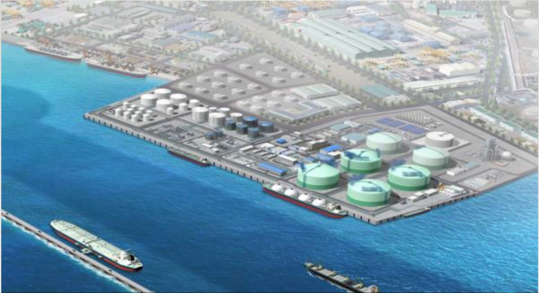
OIL&LNG Package Instrumentation Work for Ulsan North Port Liquefied Gas and Petroleum Product Terminal Korea / Completion 2024
