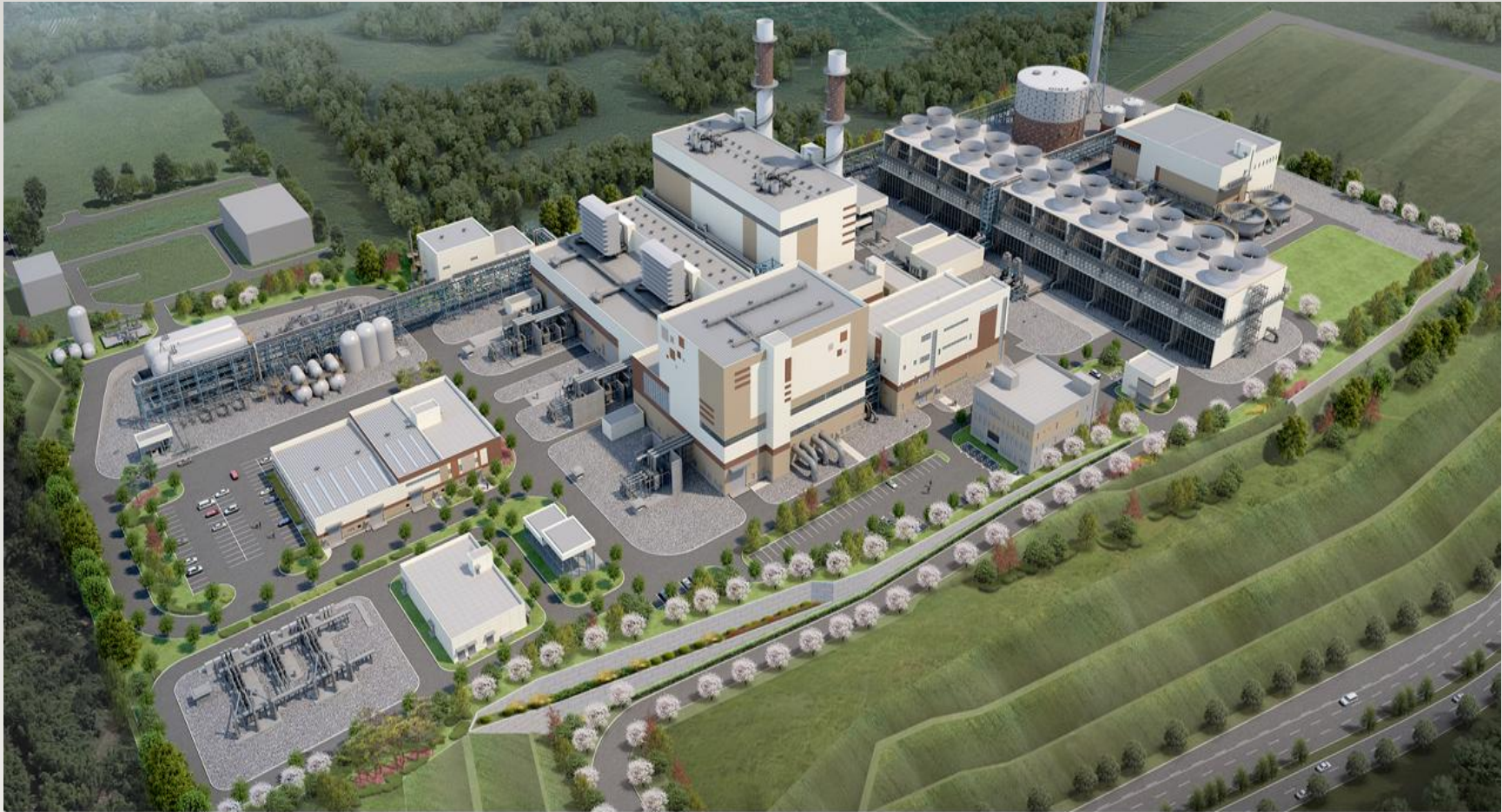
Electric Work for GPS-Combined Cycle Power Plant in Ulsan, Korea Completion 2025
